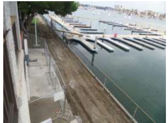
Construction going on in Anchorage
